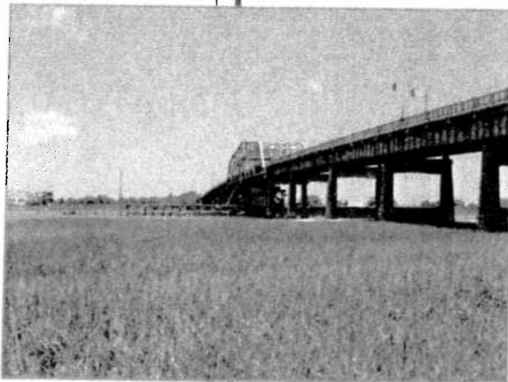
Tidal marshland beneath the bridge
