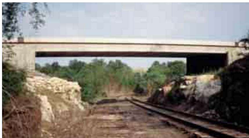
Providing a low profile while maintaining clearance over railroad tracks was a major consideration of this bridge in East Fishkill, N.Y.
