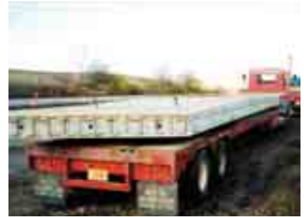
Deck panels, their post-tensioning ducts visible, arrive at the site.
