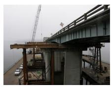
The old east approach span waits to be rolled onto temporary supports to make way for the new approach span.
