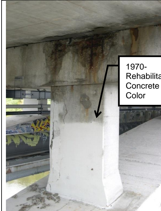
Photo SB-17.3.5 - Illustration of 1970- Rehabilitation Concrete Color - Arch rib shown (original photo is color and available from Engineer)
