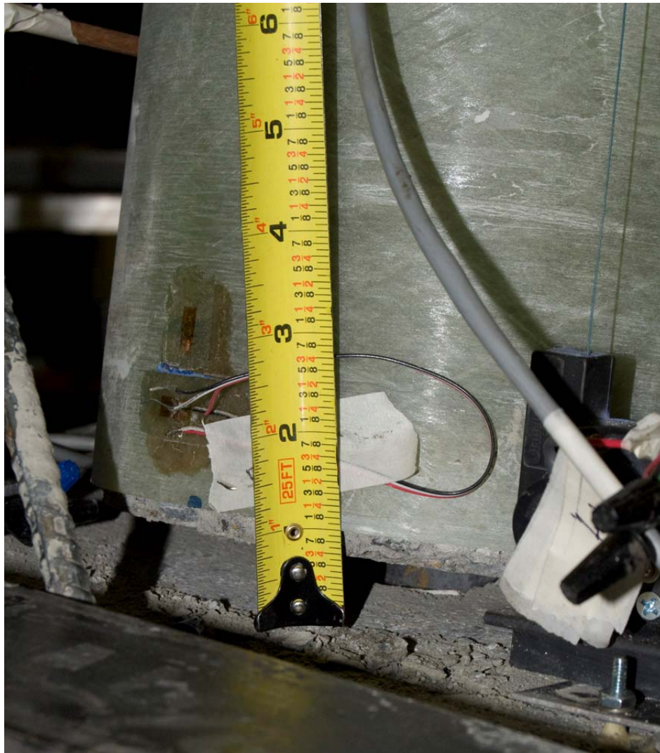
Figure 15: Specimen FRP-1 Column Rocking Mechanism
