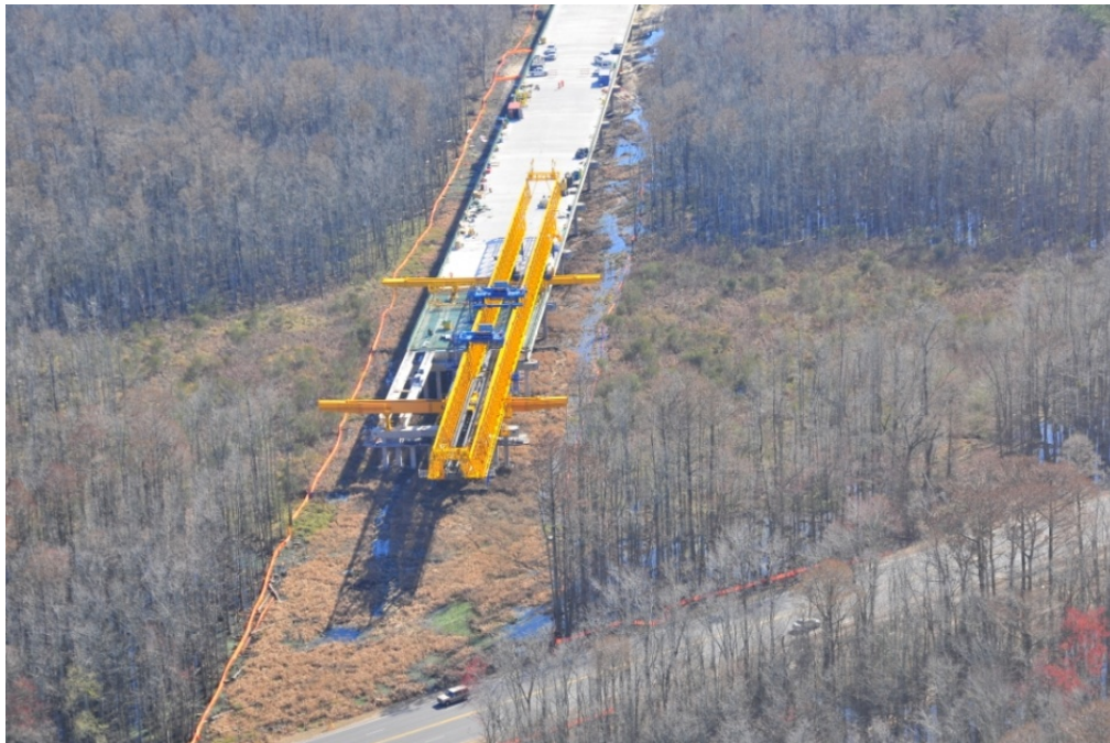
Fig. 1 Launching Gantry 1 on the south side of the project.
