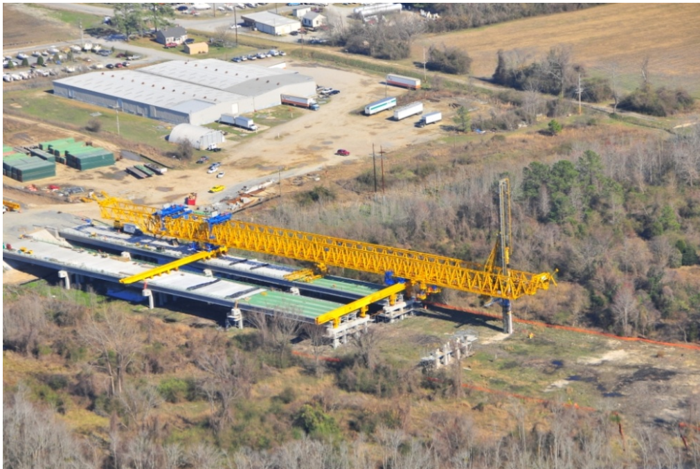
Fig. 2 Launching Gantry 2 on the North Side of the Project.
