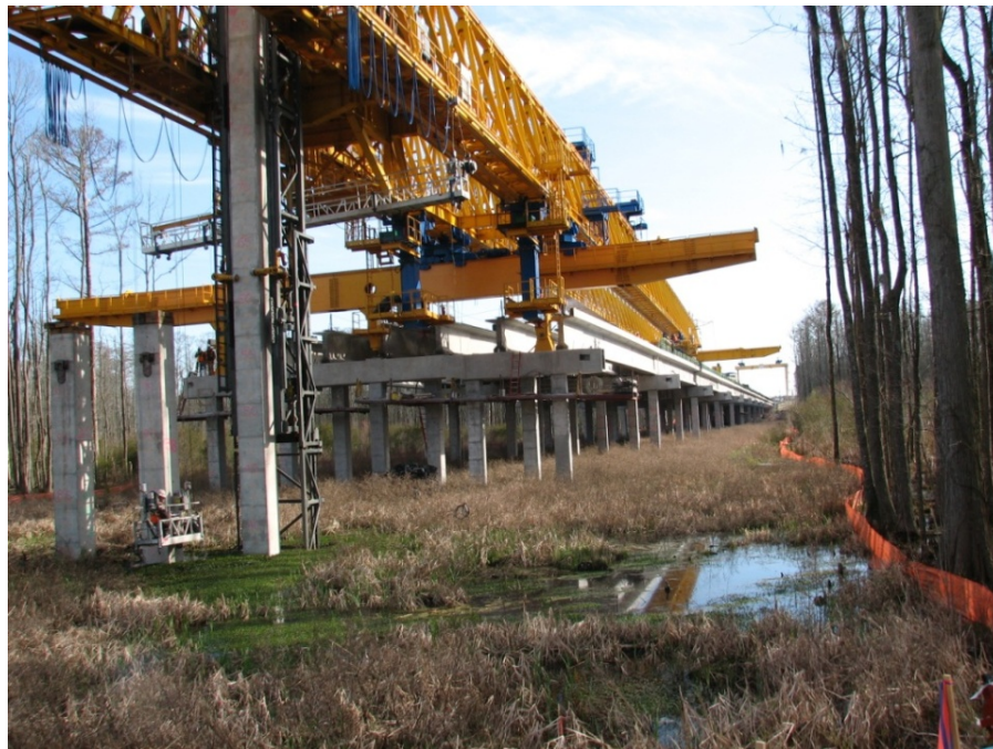
Fig. 4 Launching Gantry 1 Driving Piles in the Wetlands
