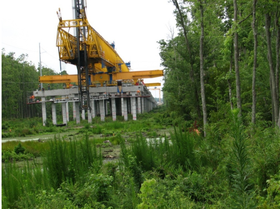
Fig. 13 Launching Gantry 1 over Wetlands
