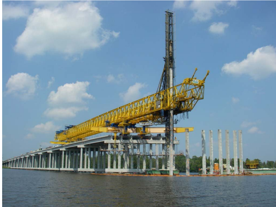
Fig. 3 Launching Gantry 2 over the Tar River
