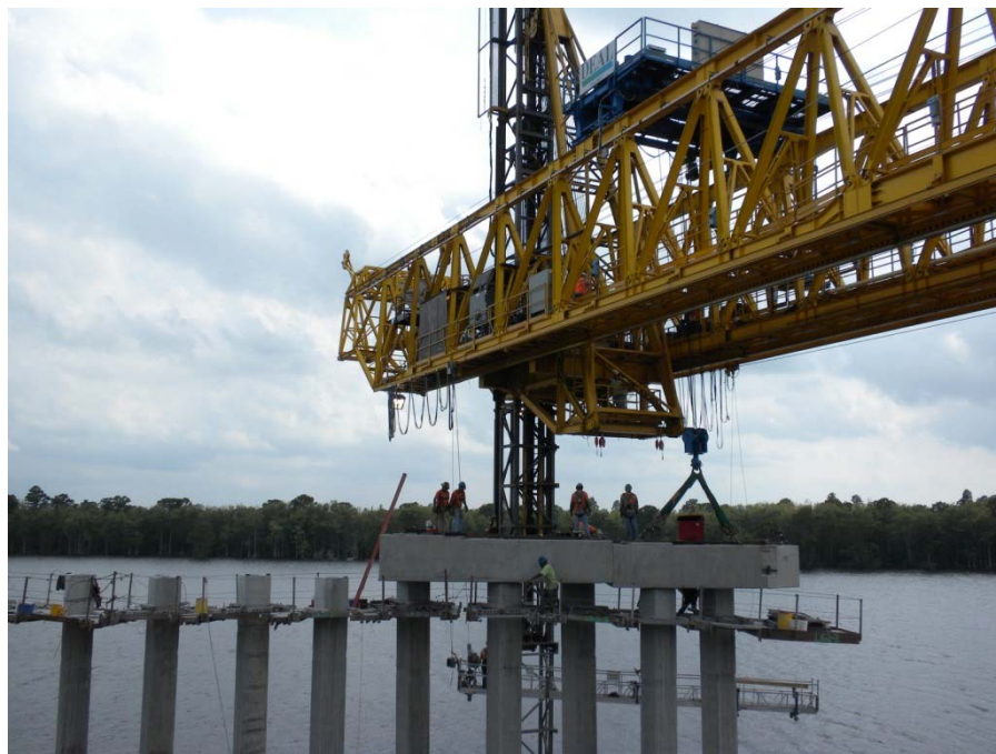
Fig. 10 Launching Gantry 1 Erecting a Precast Bent Cap
