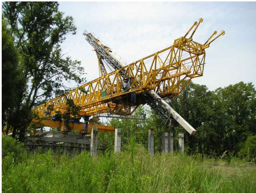
Fig. 5 Tilting Lead Rotating a Pile (US Patent 7,520,0141)
