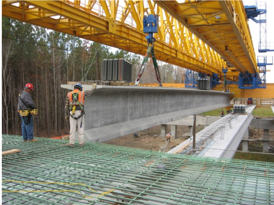
Fig.12 Launching Gantry 1 Erecting a Precast Girder
