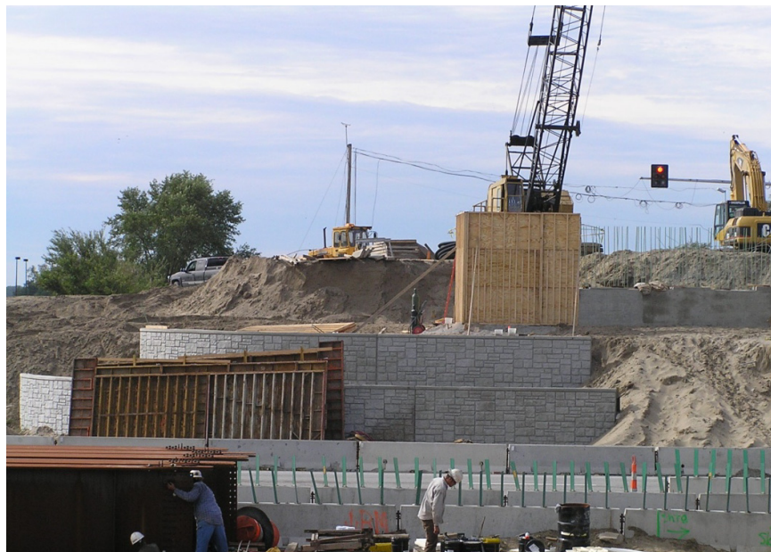
Figure 2.1. Construction of south abutment and terrace walls
