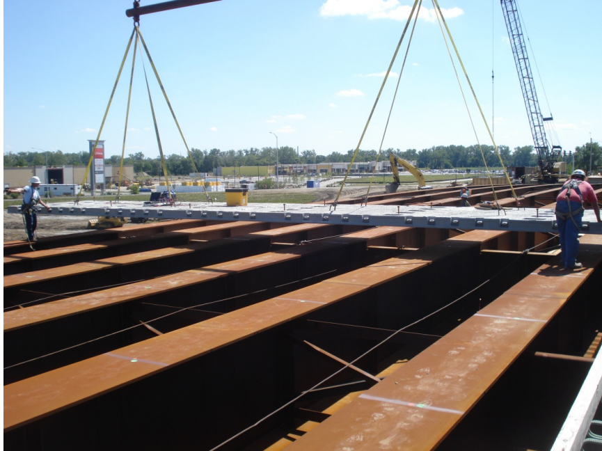
Figure 4.6. Final maneuvering of precast deck panel placement
