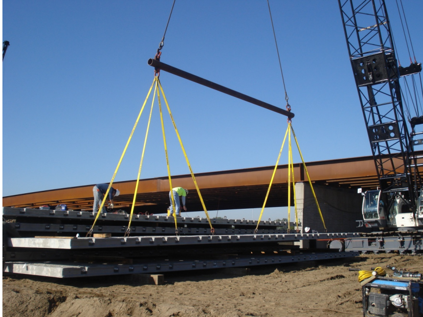
Figure 4.4. Precast deck panel in construction staging yard ready for placement
