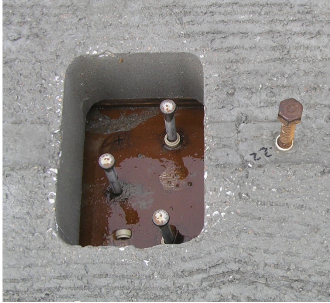
Figure 2.8. Shear stud pocket and studs
