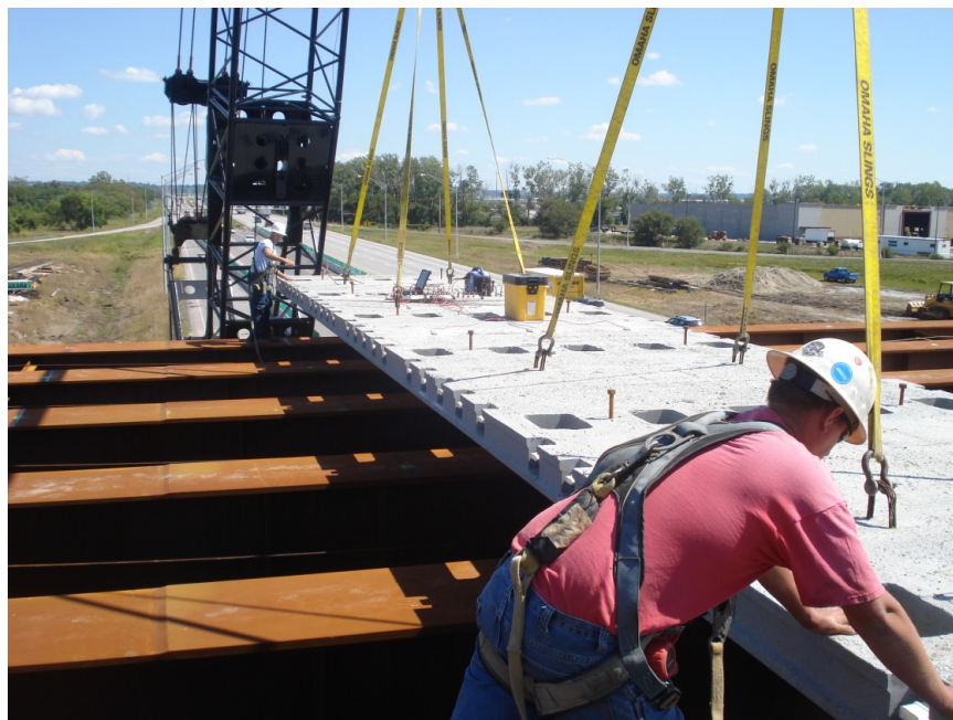
Figure 2.5. Placing precast deck panel on girders
