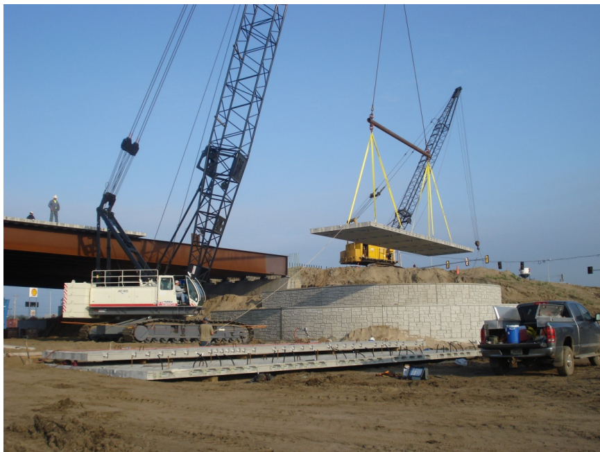
Figure 4.5. Deck panel being lifted into place
