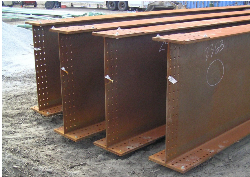
Figure 2.3. Girder ends at field splice location
