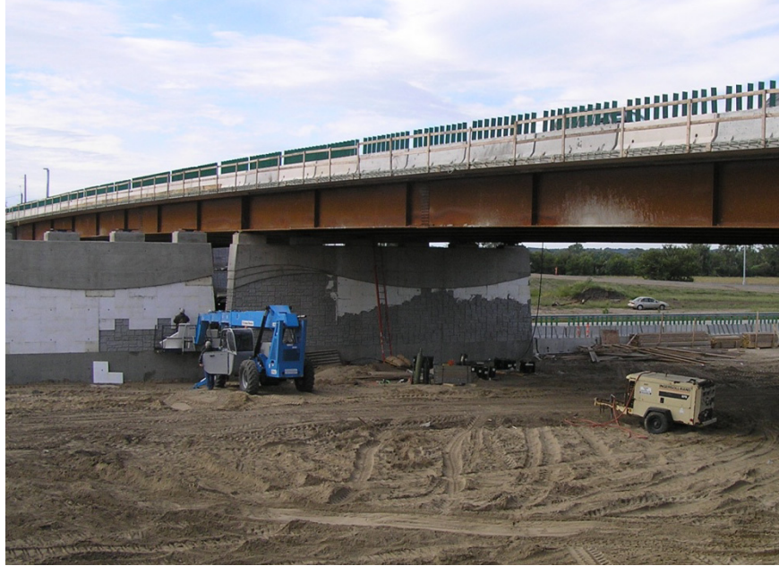
Figure 2.2. Girders on west center pier during Phase I construction
