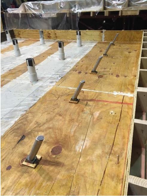
Figure 14 Inclined Bar Connection in Bridge Deck
