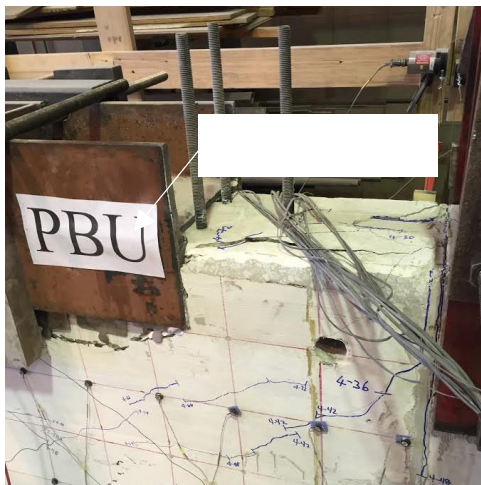
Figure 23 Cracking on barrier due to loading during Test 4
