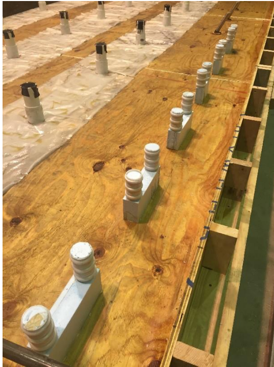
Figure 15 Pockets for U-bar Connection in Bridge Deck
