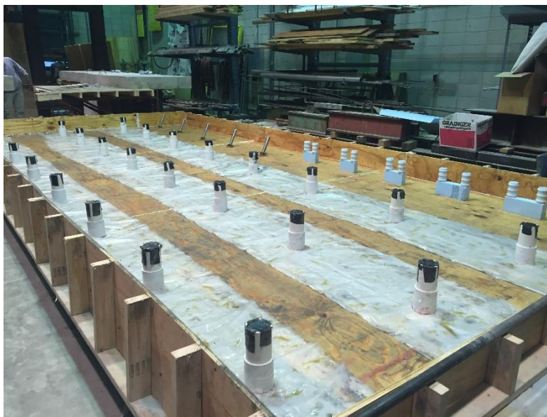
Figure 12 Concrete Beams with Deck Slab Formwork
