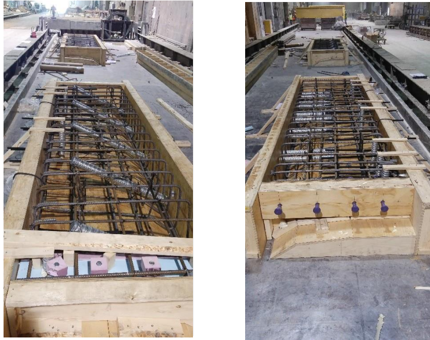
Figure 13 Precast Barrier Fabrication
