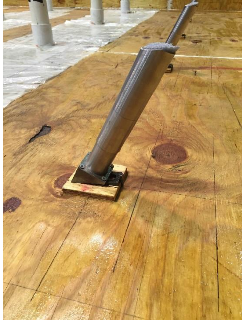
Figure 14 Inclined Bar Connection in Bridge Deck
