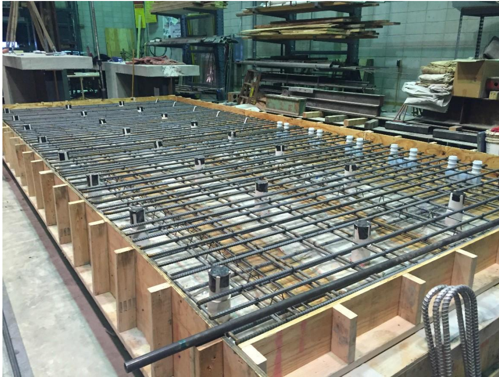
Figure 16 Bridge Deck Prior to Concrete Pour
