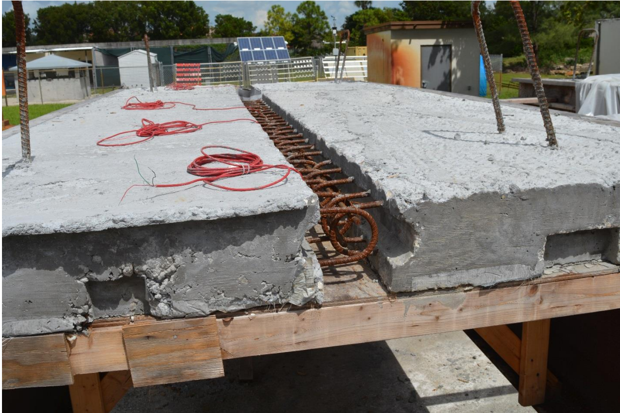
Fig. 10. Hairpin detail, note the keyway is present on this end.
