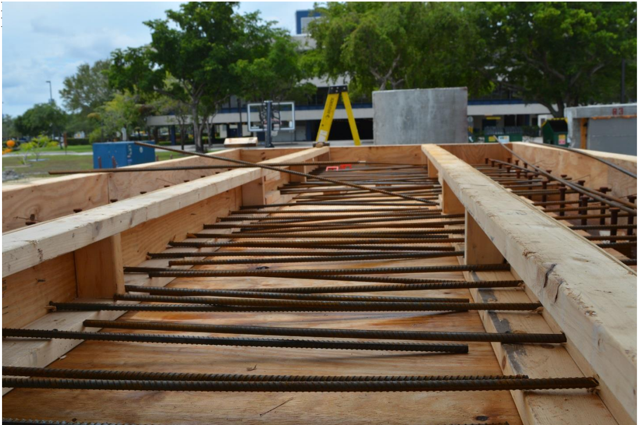
Fig. 4. Showing the Mass 14 closure detail under construction.
