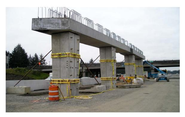
Figure 13: Grouting the Joints between Column Segments and the Column to Bent Cap
