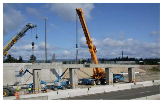
Figure 12: Precast Bent Cap Placement
