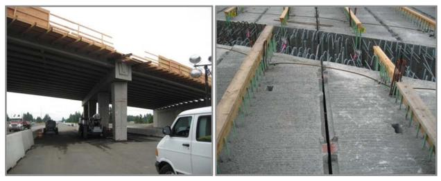
Figure 14: Placement of Precast Girders and Casting Slab Concrete
