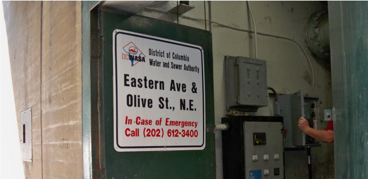
Photo 1: Entry door to pumping station (LBP door casing)
