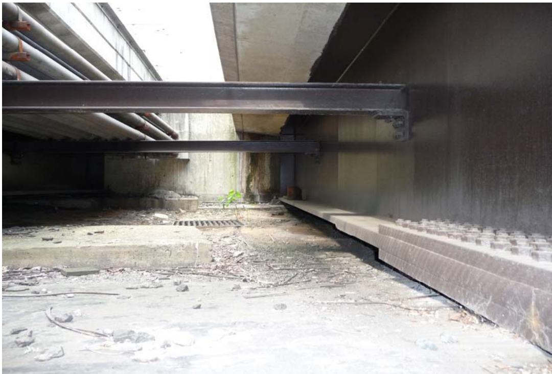
Photo No. 16- Roof Slab
