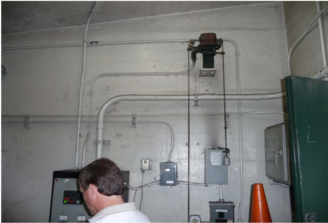
Photo No. 5- Motor Room, Walls
