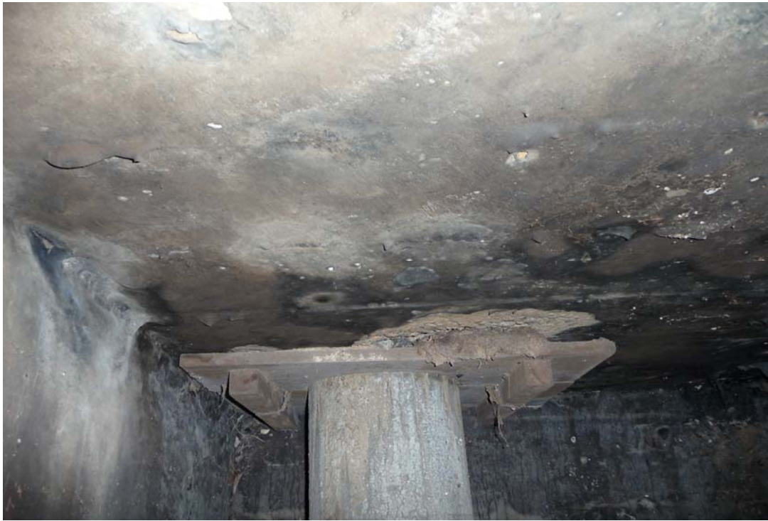
Photo No. 15- Sump Room, Ceiling at Float Pipe
