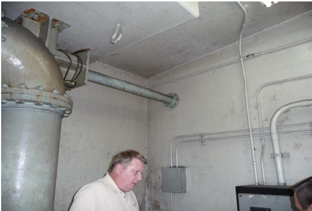
Photo No. 4- Motor Room, Walls
