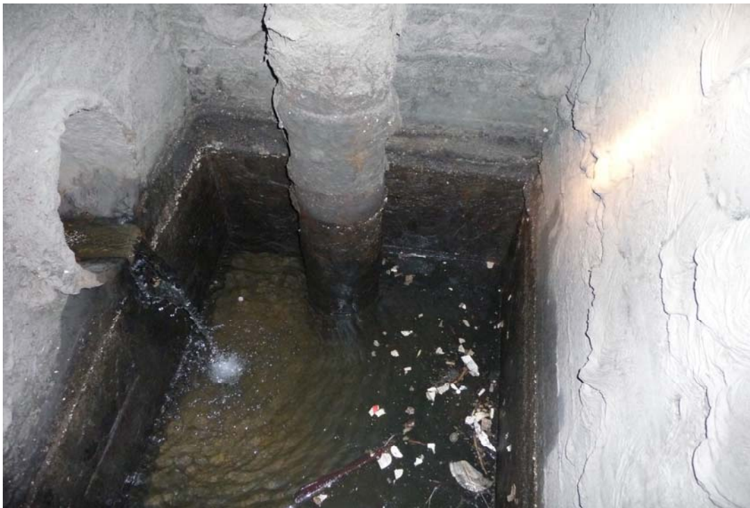
Photo No. 14- Sump Room
