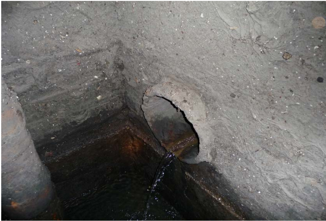
Photo No. 13- Sump Room
