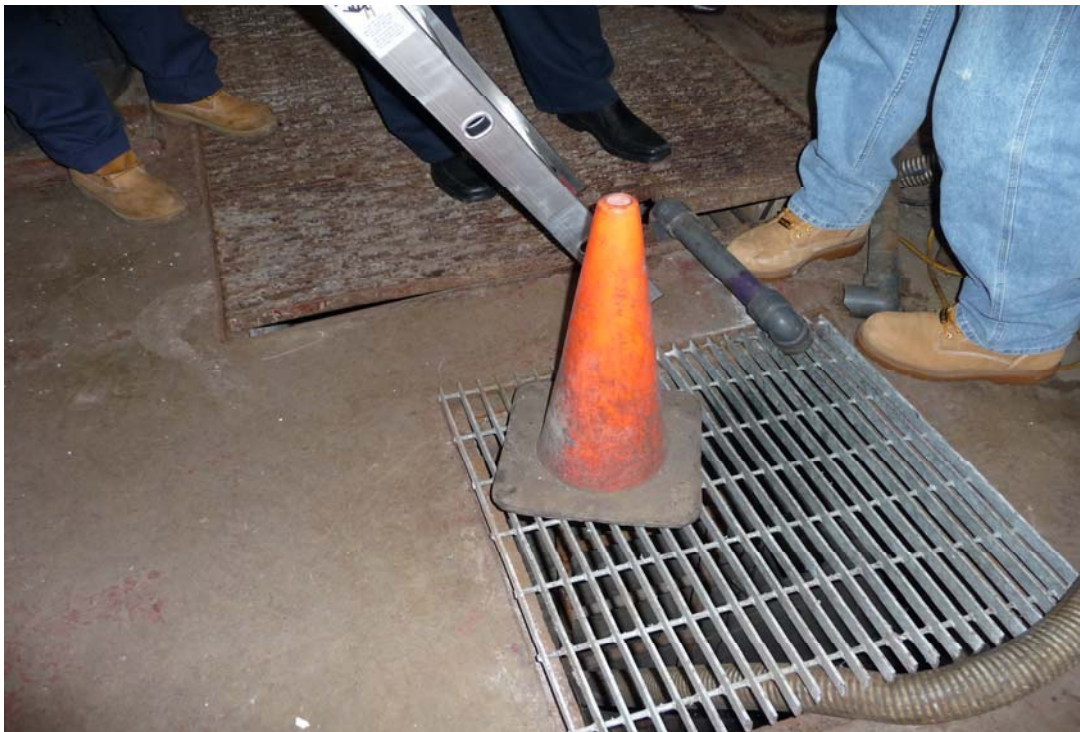
Photo No. 6- Motor Room, Floor
