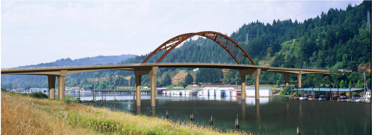
Figure 1. Photo-simulation of the 5-span replacement bridge
