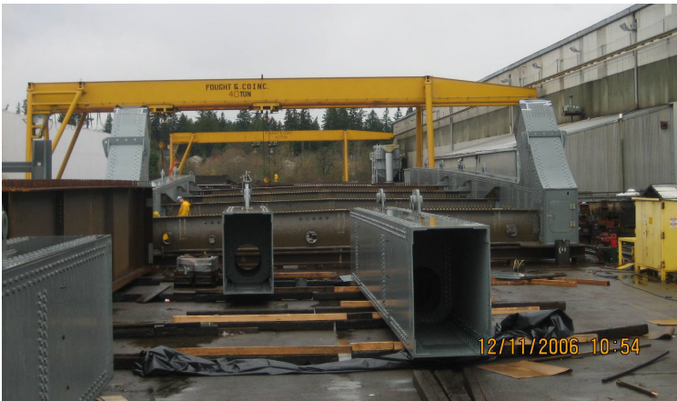
Figure 11. Installation of permanent casing for drilled shafts
