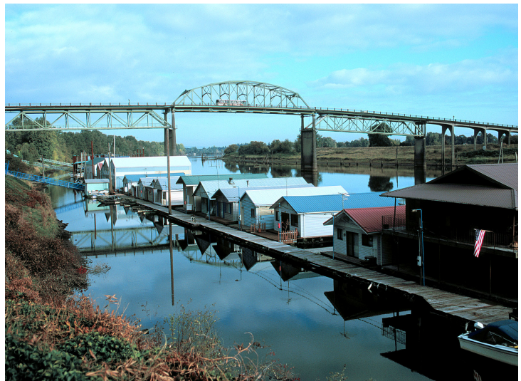
Figure 2. Existing Sauvie Island Bridge
