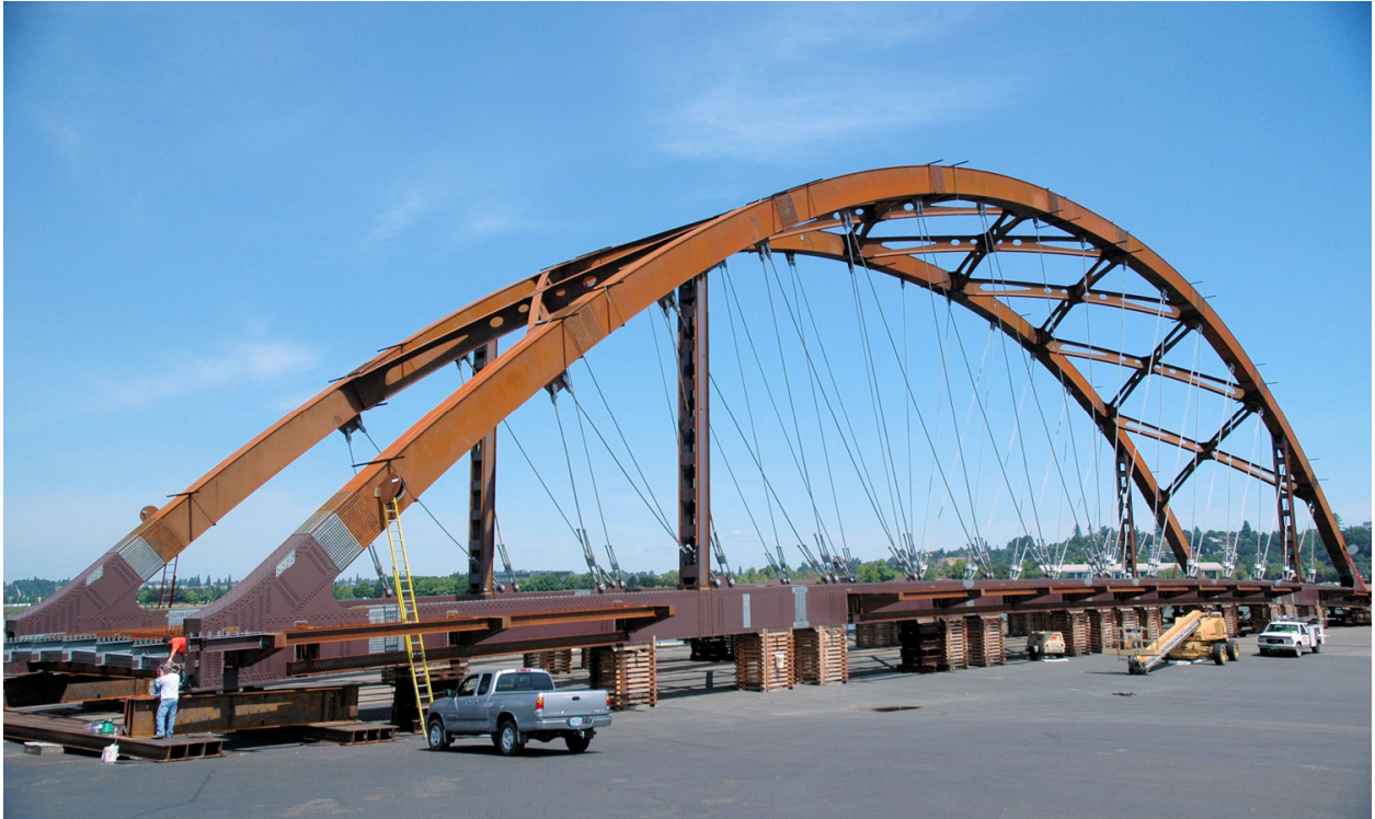
Figure 12. Completed Span on Port of Portland Dock
