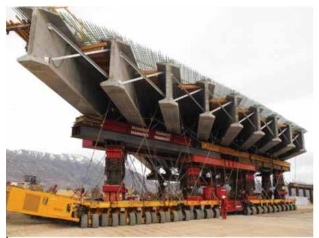
During lifting and transport, as any support would move relative to the other three supports a displacement would result where the diagonal string lines intersect in the middle of the spans. Active adjustments were made to the supports during transport.
