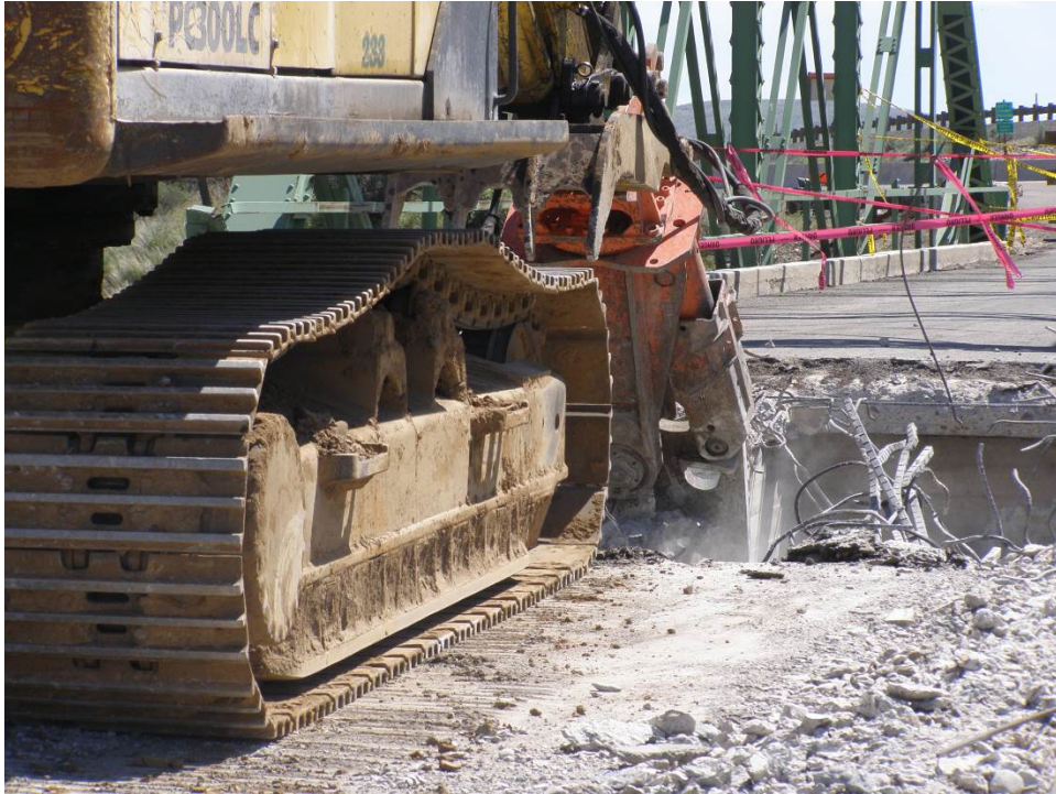
Figure 19. Closeup of demolition of approach to bridge 0700.
