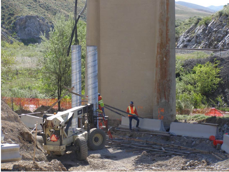
Figure 23. Installation of corrugated metal pile spacers for building the substructure and MSE retaining wall.
