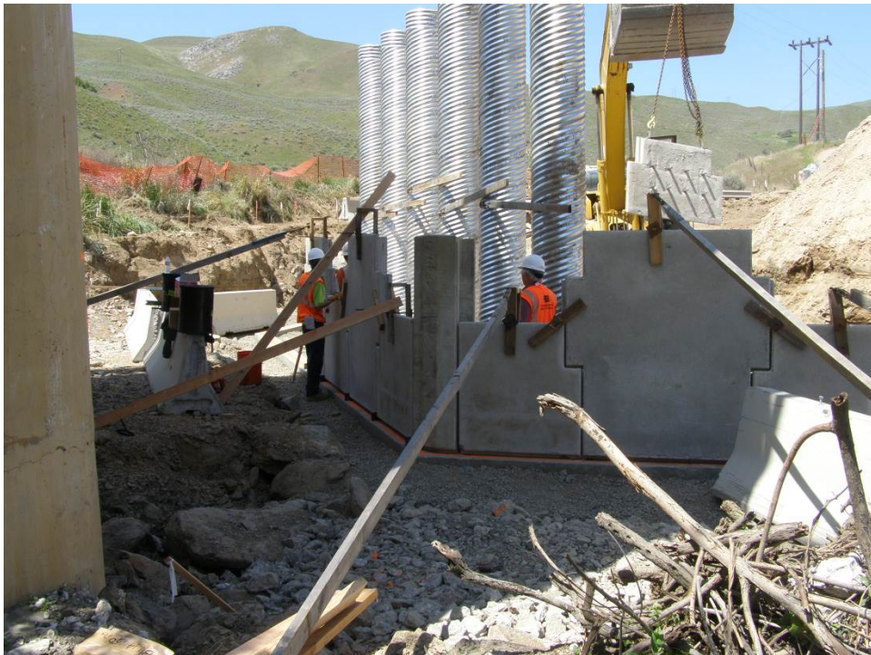
Figure 24. Installing MSE retaining wall (side view).
