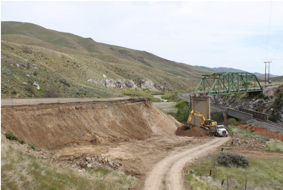
Figure 20. Excavation for building the substructure and installation of MSE wall.
