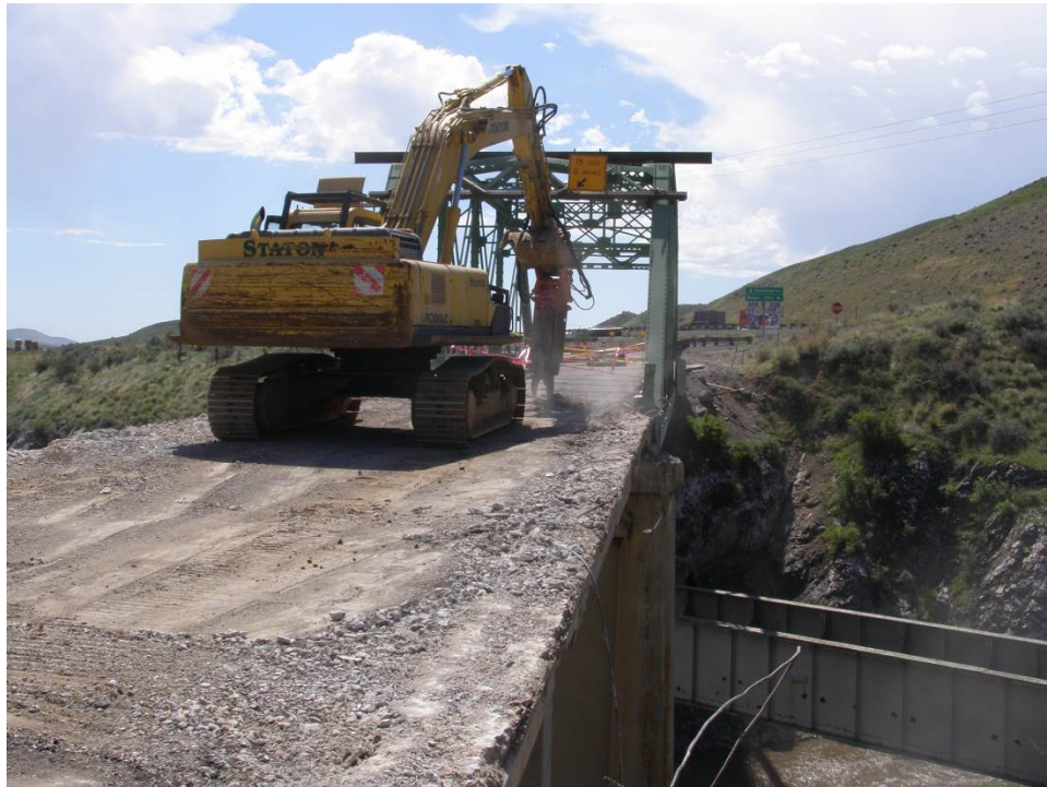
Figure 17. Demolition of approach to bridge 0700.
