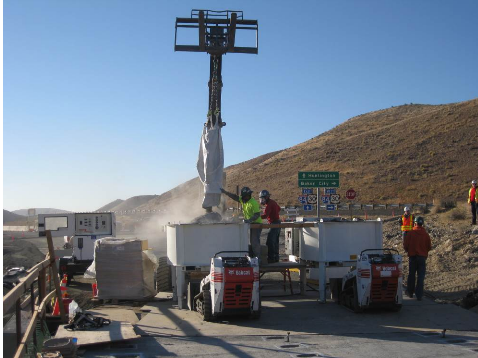
Figure 47. UHPC aggregate being put in the mixer.
