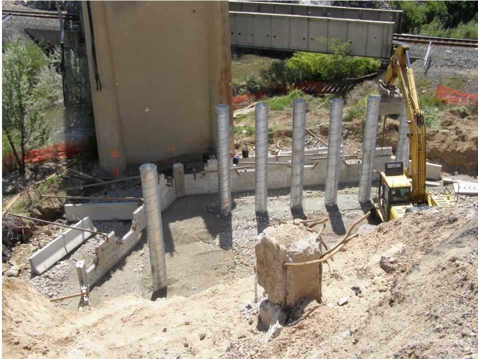
Figure 26. Installing MSE retaining wall (top view).
