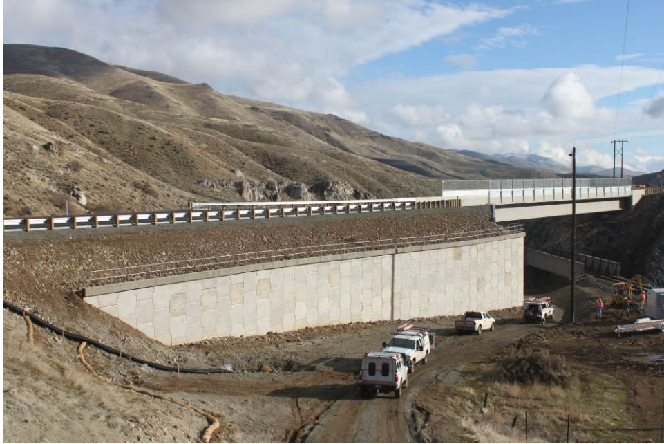
Figure 57. Overview of bridge 21252 after completion.
