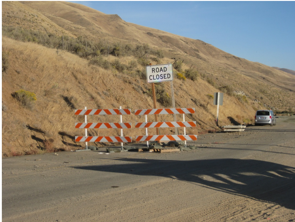
Figure 59. Closure of Old US30 at the north end of the project.
