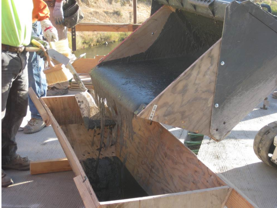
Figure 51. Placing the UHPC in the shear pockets.
