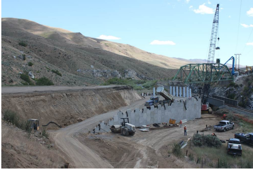
Figure 27. Backfilling MSE retaining wall (long view).
