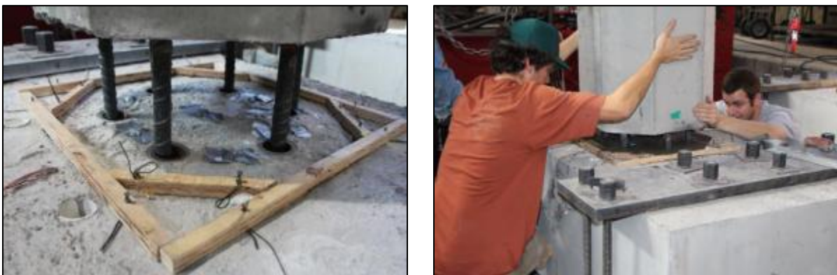
Figure 2-14. Grouting operation for GGSS-2.
