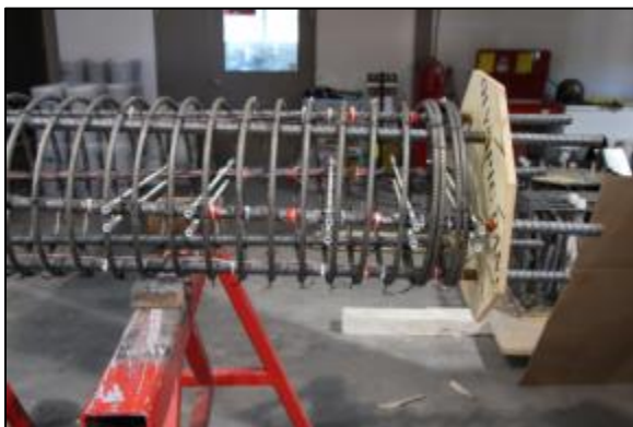
(a) Column cage with projecting bars.
