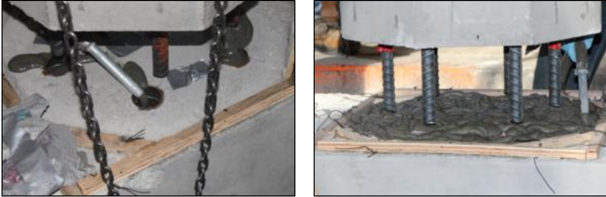
Figure 2-37. Grouting operation for FGSS-2.
