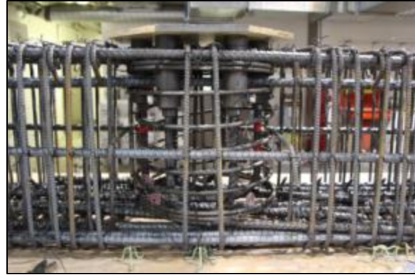
(b) FGSS placed within cap beam.
