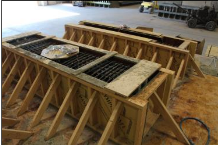
Figure 2-36. FGSS-2 precast components inside concrete forms.
