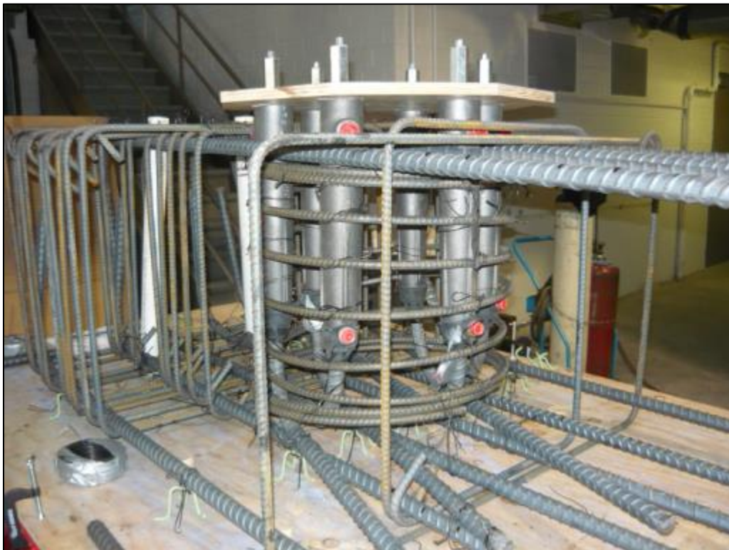
Figure 2-10. GGSS-2 precast footing core rebar cage.
