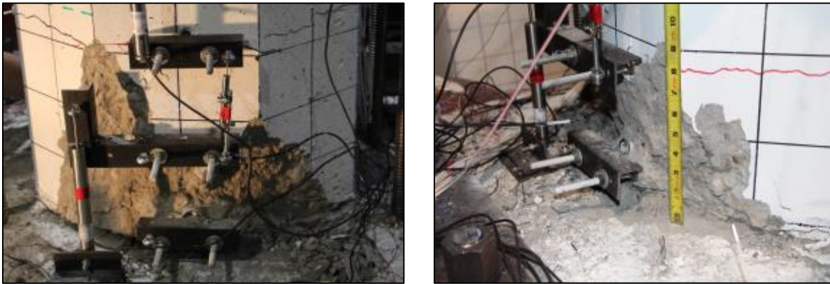
(b) Damage state at 6% drift ratio: cracks, spalling, and yield penetration.
