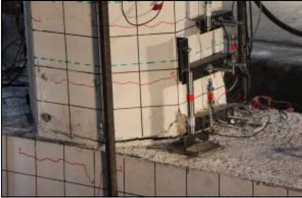
(a) Bed grout opening at 3% drift ratio (peak).
