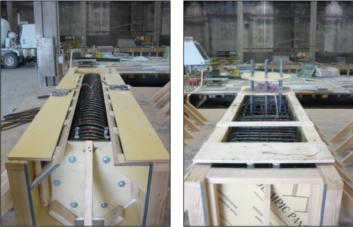
Figure 2-30. FGSS-1 precast components inside concrete forms.
