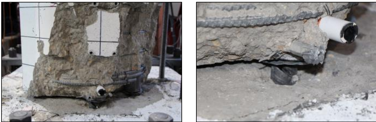
(c) Damage state at 9% drift ratio: spalling, exposed rebar cage, and fractured bar.
