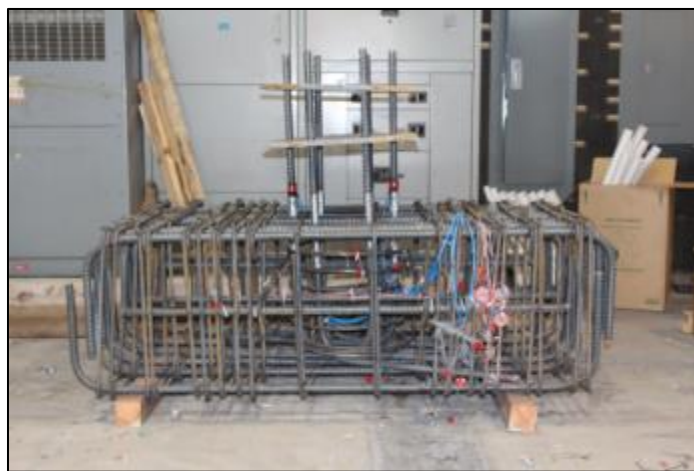
(b) Footing rebar cage.
