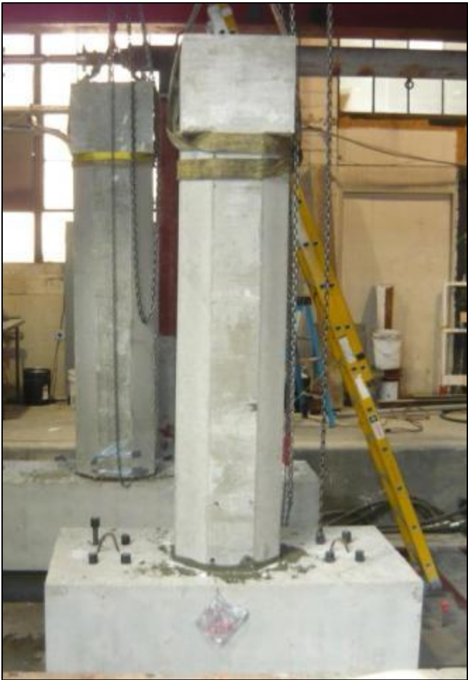
Figure 2-8. GGSS-1 in the final position.
