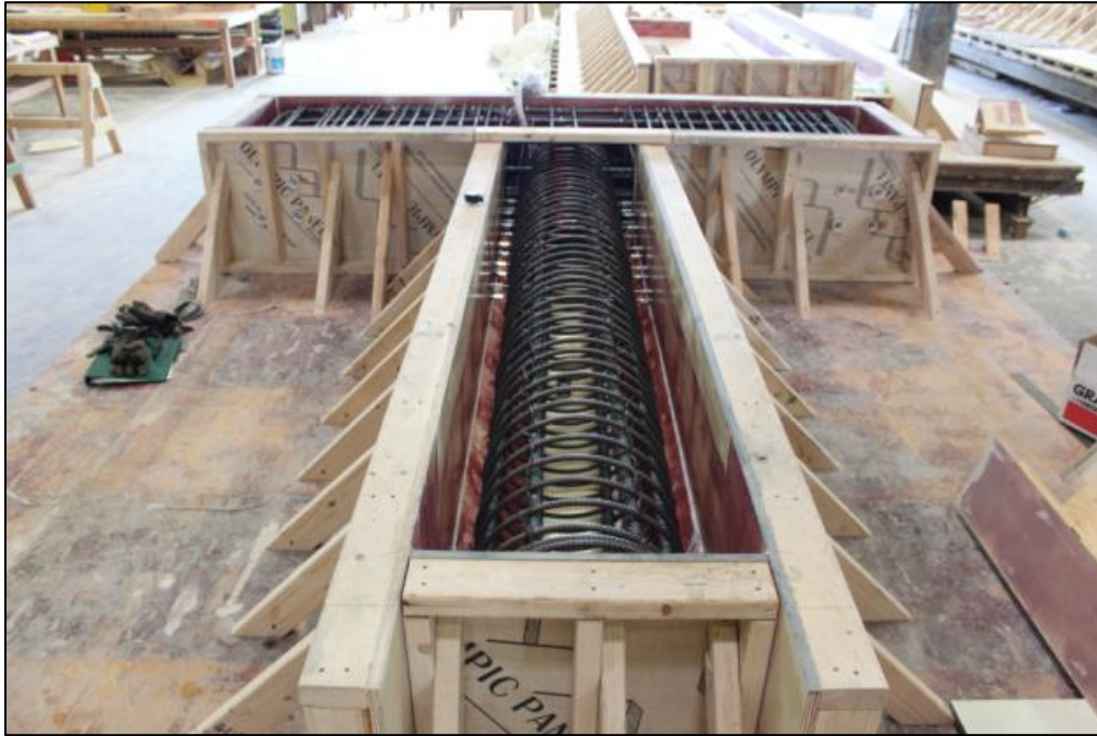
Figure 2-48. FGSS-CIP rebar cage inside concrete form.
