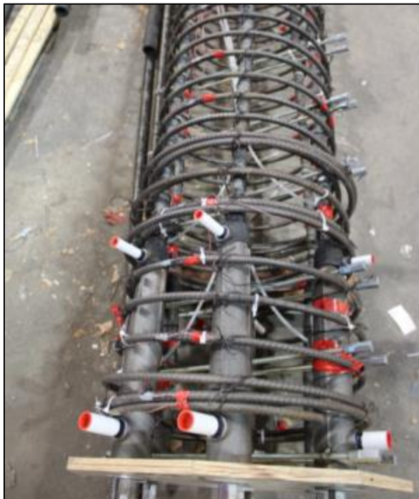
(a) LVDT all-thread rods attached to rebar cage
