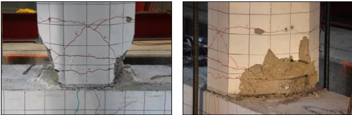
(b) Damage state at 7% drift ratio: cracks, spalling, and exposed spiral.
