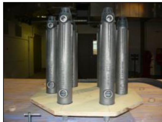
(b) GGSS fastened to template for the footing.
