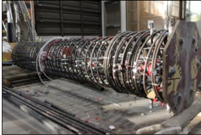
(a) Column rebar cage.
