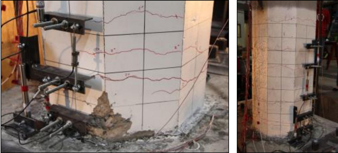
(a) Damage state at 3% drift ratio: cracks and spalling.
