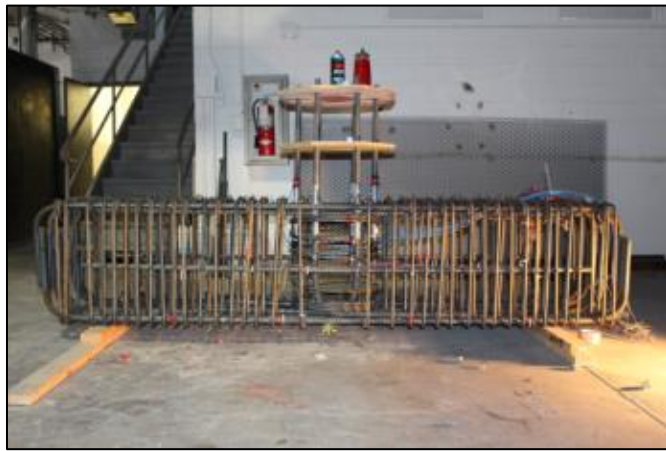
(b) Cap beam rebar cage.
