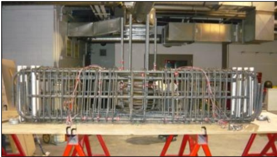
(b) Cap beam rebar cage.
