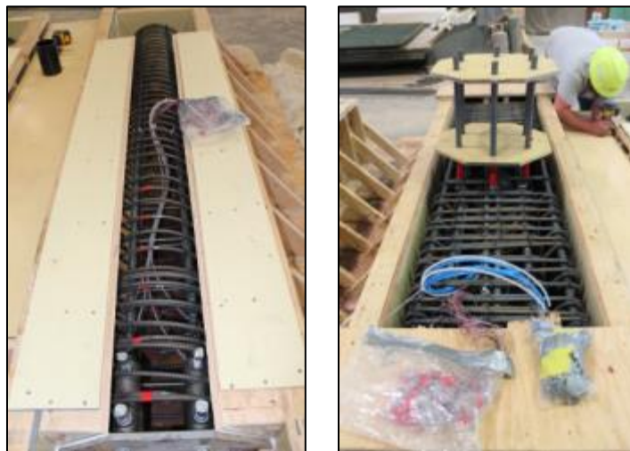
Figure 2-43. FGSS-3 precast components inside concrete forms.
