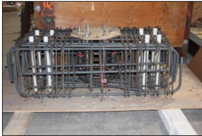
(b) Footing rebar cage.
