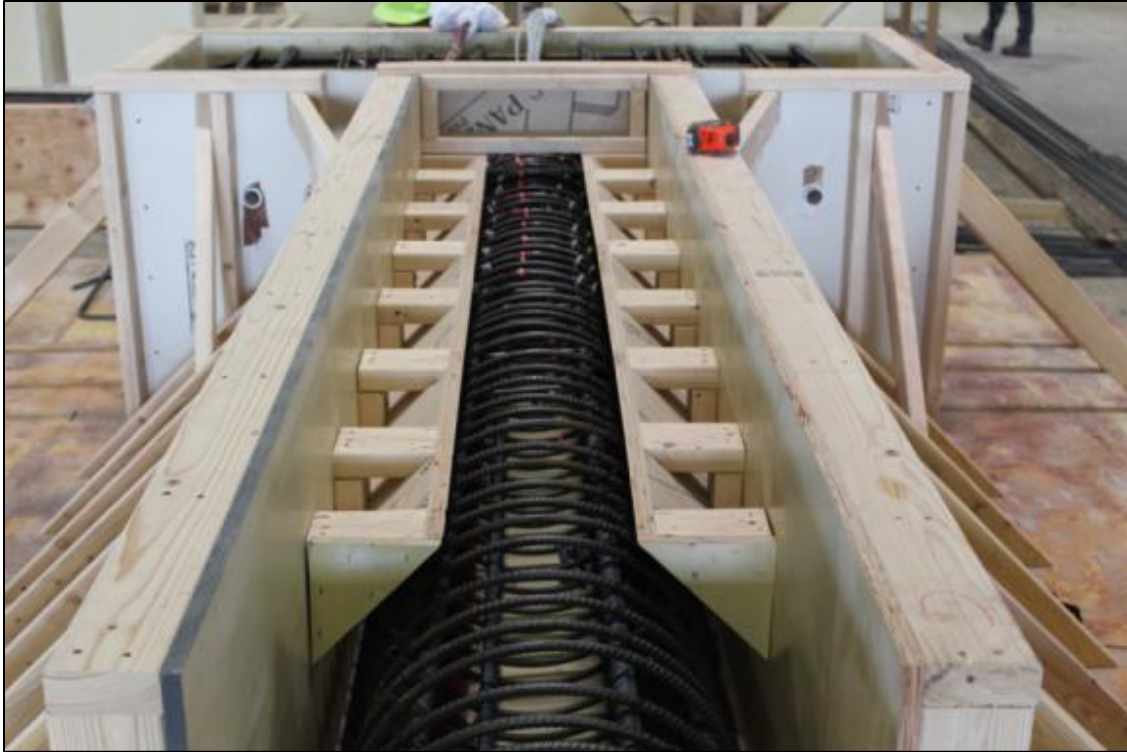
Figure 2-25. GGSS-CIP rebar cage inside concrete form.
