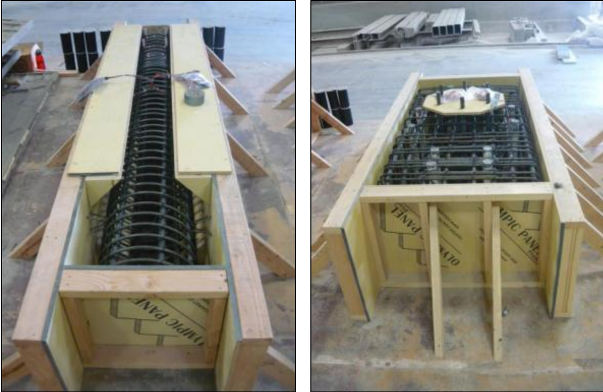
Figure 2-6. GGSS-1 precast components inside concrete forms.
