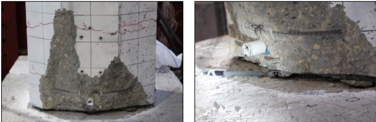
(b) Damage state at 8% drift ratio: cracks and spalling, fractured bar, and exposed rebar cage.
