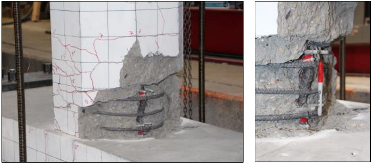
Figure 4-57. Damage state for FGSS-CIP at end of test: cracks and spalling, rebar buckling and fracture.
