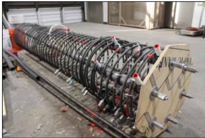
(a) Column rebar cage.
