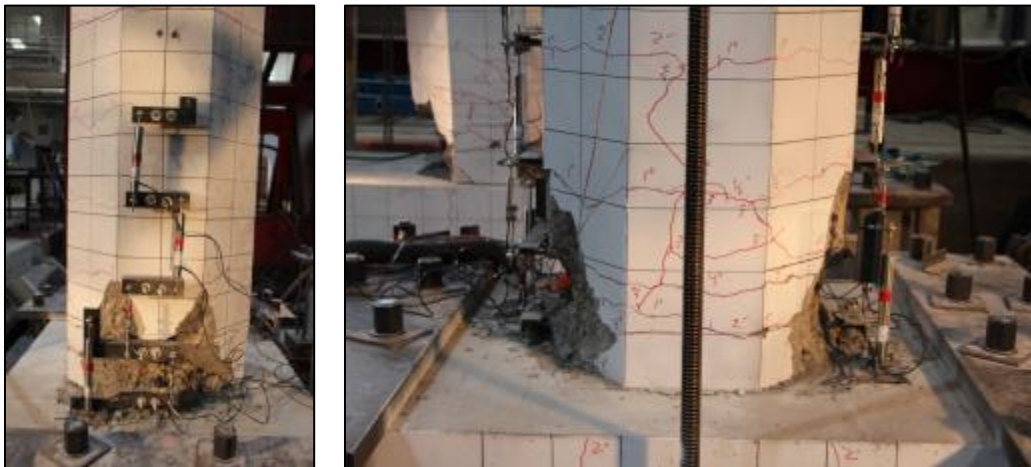
(b) Damage state at 6% drift ratio: spalling and inclined cracks.
