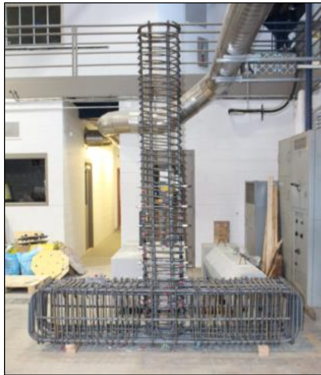
(b) Rebar cage ready to cast concrete.
