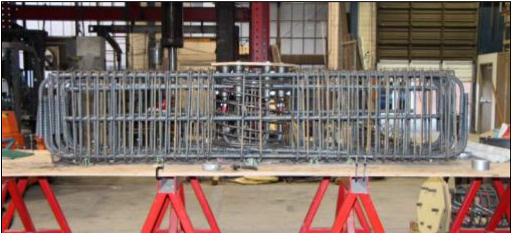
(b) Cap beam rebar cage.
