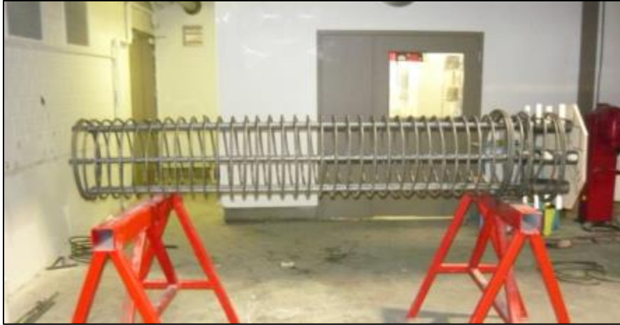
(a) Column rebar cage.
