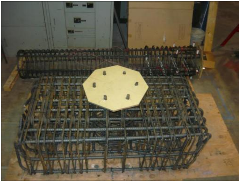
(b) Column and footing rebar cages.
