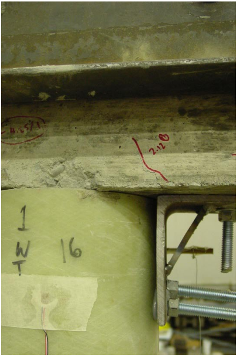
(a) Northern corner
