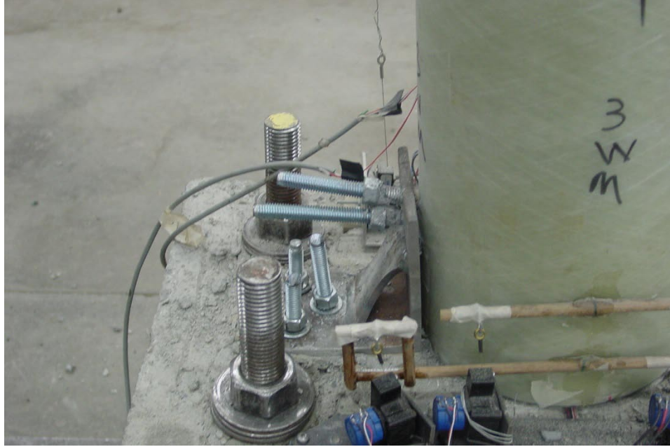
Figure 5.2.31: Bolts fixing angles to lower column-segment of northern column of specimen F-FRP3-S pulled out of position after 3.80 in. displacement level
