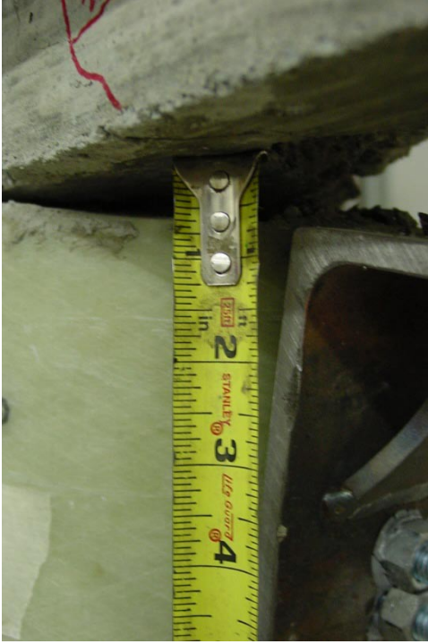
(a) Column-beam interface of northern column
