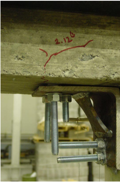
(b) Southern corner
