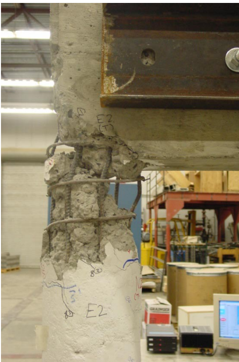
(c): Top of Column S
