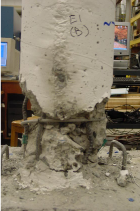
(a): Bottom of Column N
