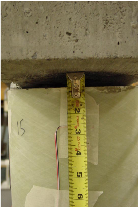
(c) Column-beam interface of southern column
