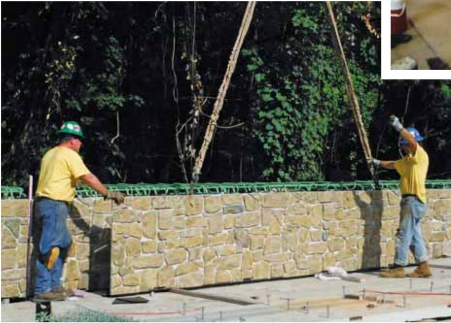
A unique design was developed that utilized architecturally treated precast panels resembling natural stone construction to blend in with the historic nature of the area. The parapet panels served as permanent stay-in-place forms for the cast-in-place concrete core between the panels.
