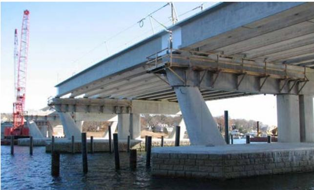
**Figure 20. Westbound bridge piers are shown in various stages of completion.**
