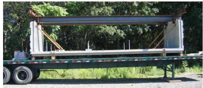
**Figure 8. Cofferdam section delivered to the project site and fitted with lifting beams.**
