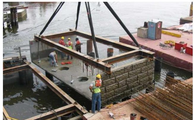
**Figure 9. Precast cofferdam section being hoisted into place.**
