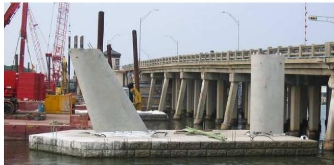
**Figure 12. The first precast pier columns.**
