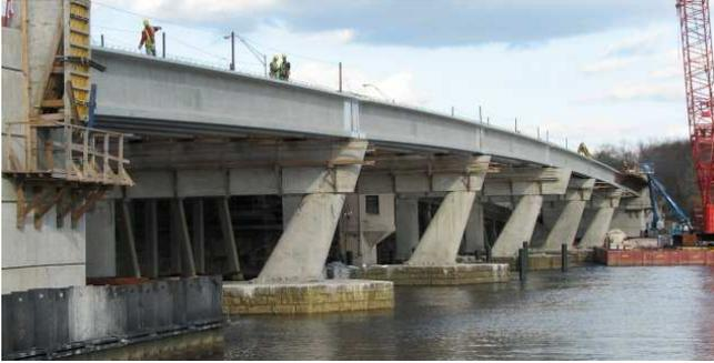
**Figure 19. Piers 1EB through 5EB have been completed and the bulb tee girders erected.**
