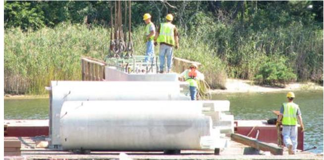
**Figure 11. Precast pier columns and a cap beam are being prepared for erection.**
