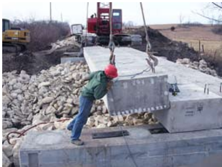
Figure 11 - Placement of box girders at the Madison County site
