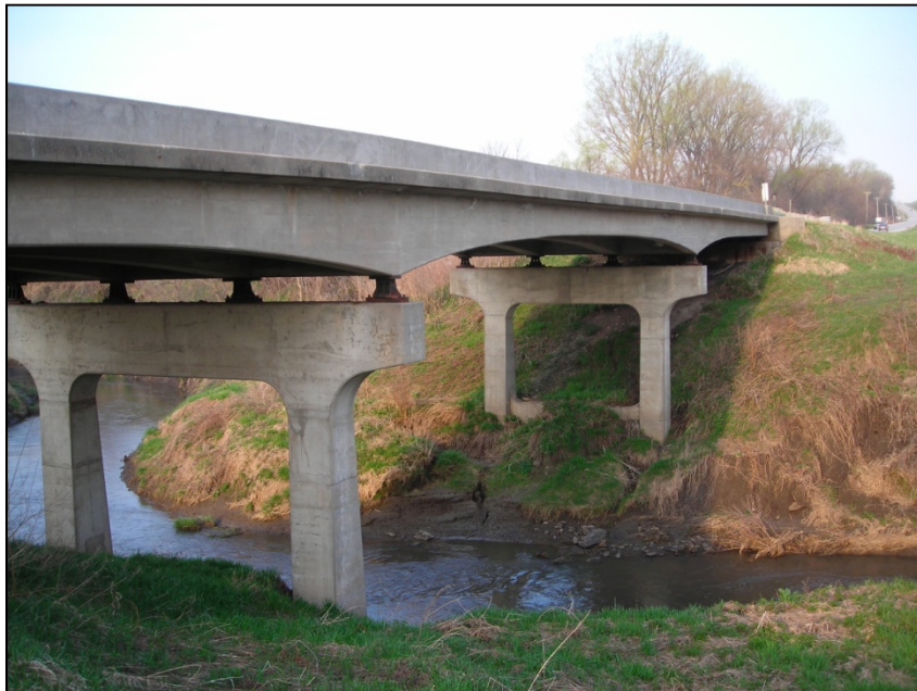
Figure 1. Existing US 6 bridge over Keg Creek.
