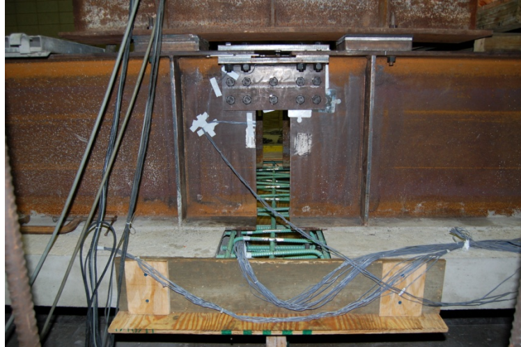
Figure 10. Full scale lab test specimen prior to placing UHPC concrete
