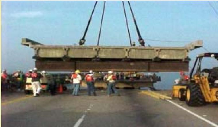
incentive/disincentive clause. Work was completed in the summer of 2002. With its 7½-inch concrete slab cast on precast prestressed concrete girders, the new span was built on a barge on the north shore of Lake Pontchartrain
