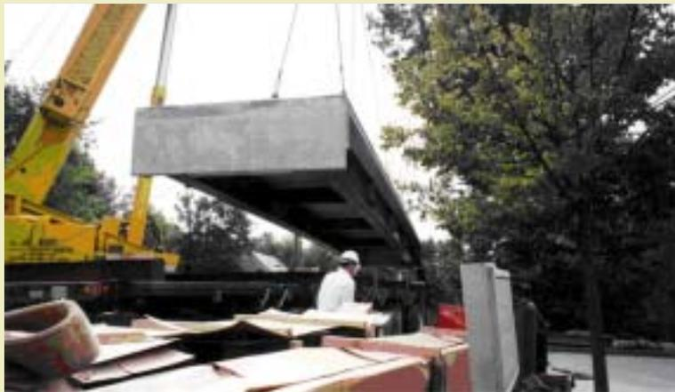
and transported to the site on trucks and lifted into place by a crane. Each of three prefabricated units consisted of two rolled beams with a precast reinforced concrete bridge deck. In place, the three units provided a complete superstructure except for
