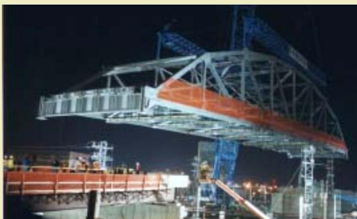
The 320-ft. long, 850-ton prefabricated truss center span was constructed over several months next to the active rail lines and then lifted into place on an early Sunday morning in May by a single high-capacity crane owned by Lampson International LLC. The crane lifted the entire truss span 65 ft. and moved it 100 ft. to its final position.
