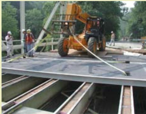
after placement, the forklift could start at one end of the bridge, set a panel, and then move onto that panel to set the next. Work on the new deck was completed in 2001.
