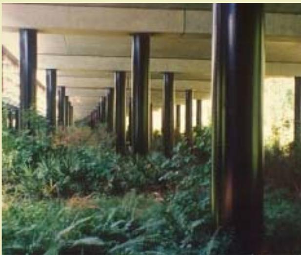
shallow 2 ft. 5 in.-deep precast deck panel superstructure. Except for touch-up painting of the steel piles, all work was completed from the top with no activity on the creek bed below.
