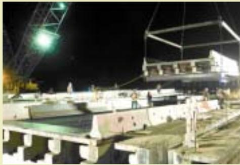
outside the travel lanes of the existing bridge, install new precast prestressed bent cap shells on the piles, and pour concrete and then prestress the caps. Then crews start from the abutment using a barge-mounted crane to sequentially replace the superstructure. Two 50-ft. spans totaling 100 ft. of
