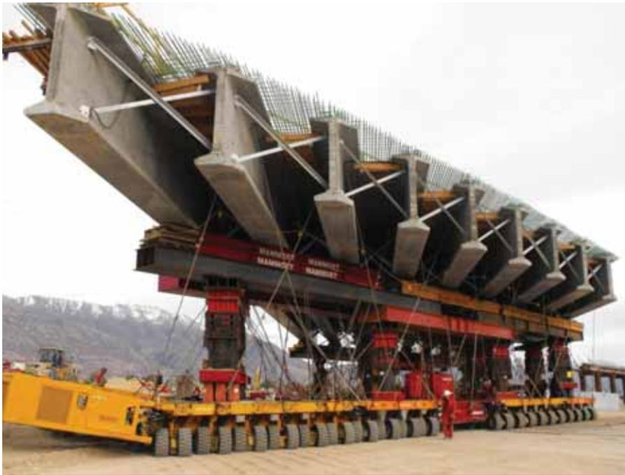
During lifting and transport, as any support would move relative to the other three supports a displacement would result where the diagonal string lines intersect in the middle of the spans. Active adjustments were made to the supports during transport.
